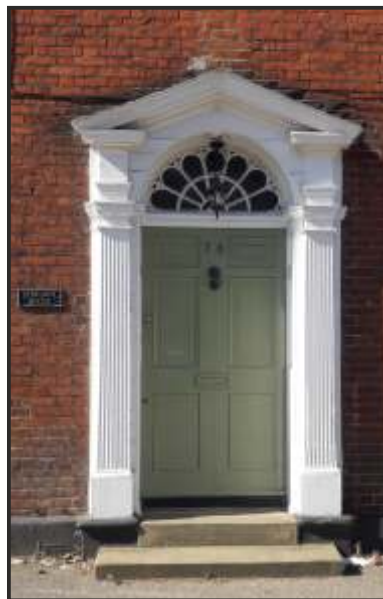
Door case to Sebright House with pediment and fanlight
