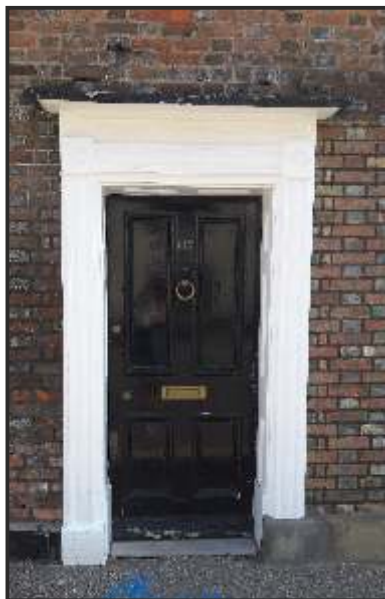
Door case to 117 High Street
