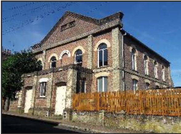
Markyate Methodist Church, Wesley Road (this view from Albert Street).
