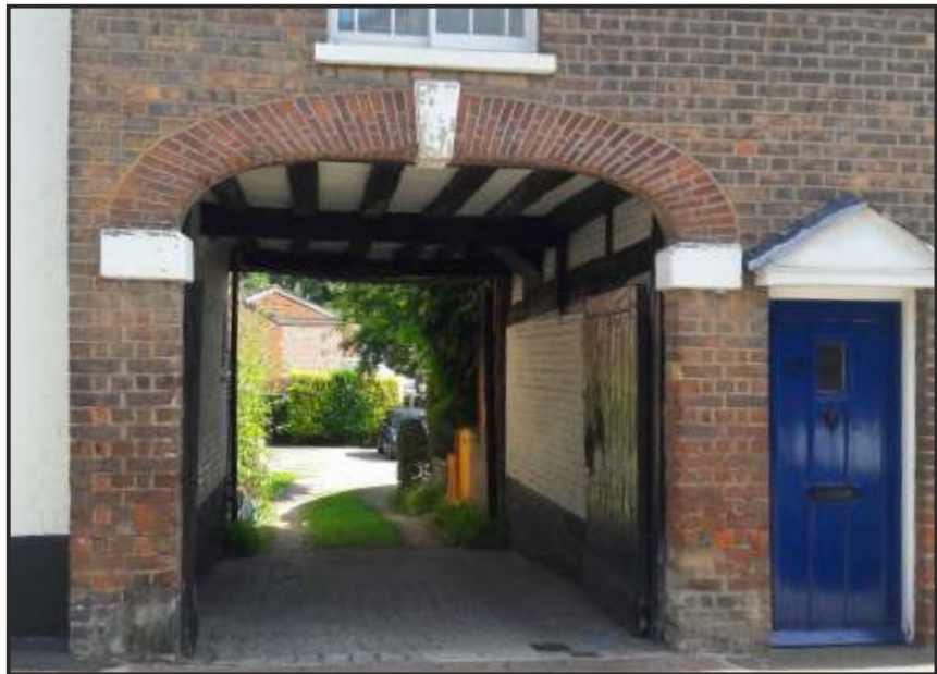
Timber frame visible in carriage arch to 59 High Street
