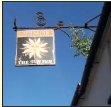
Retained wrought iron bracket and The Sun Inn sign
