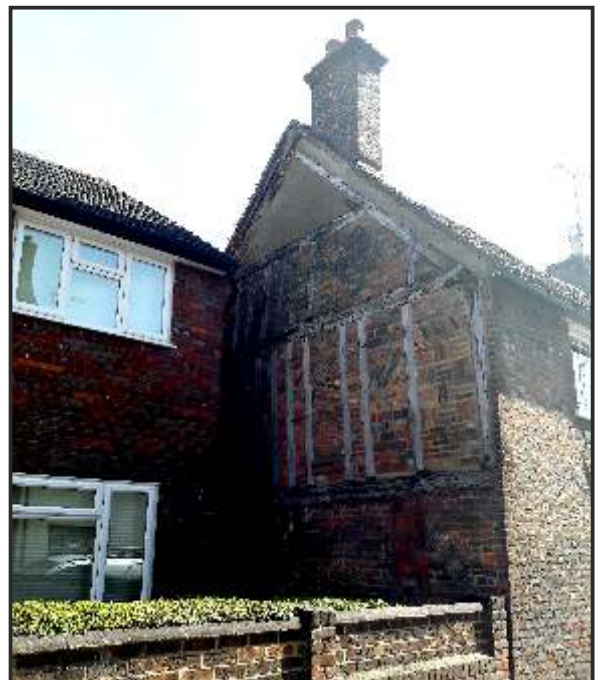
Timber frame to gable end, 117 High Street
