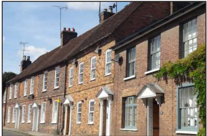
Satellite dishes to front elevations of properties along Pickford Road
