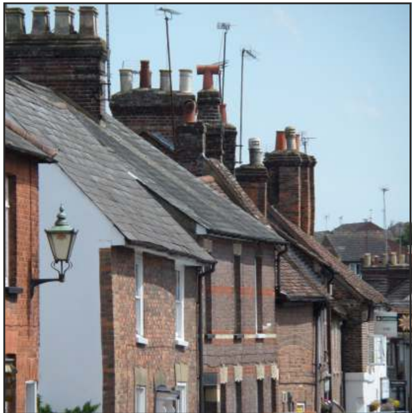
Markyate High Street roof scape, east side looking south
