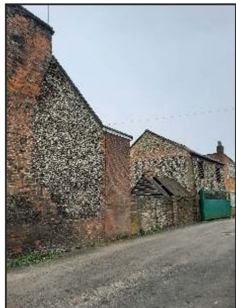
Flintwork to side wall of 52 High Street and outbuilding to rear
