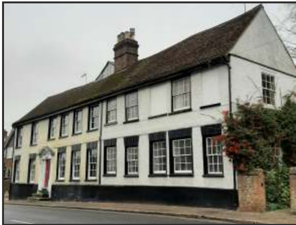
Sash windows to The Grange
