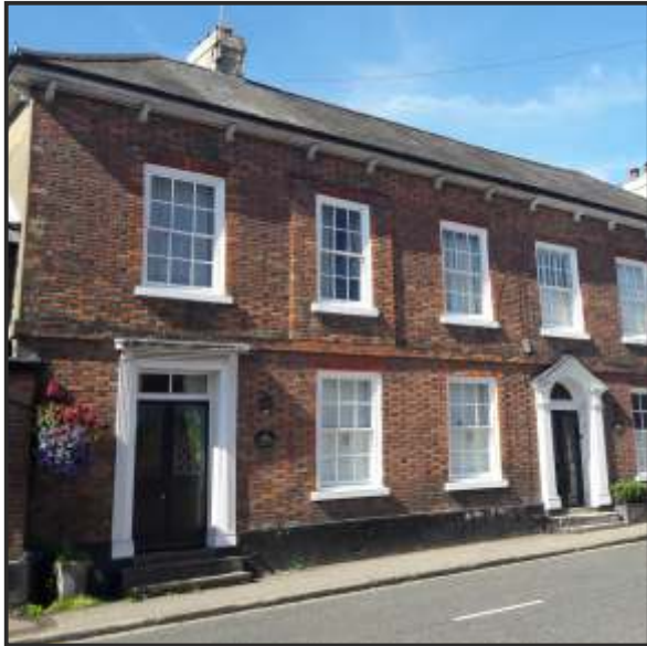
Village Place, red brick laid in Flemish bond with dark brick headers
