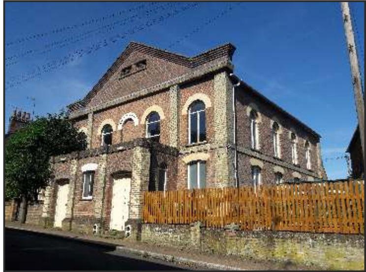
Markyate Methodist Church, Albert Street
